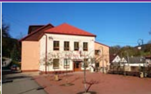
School building, square
